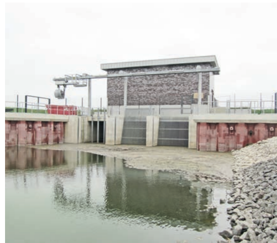
Pump Station Luneplate VP 900 vertical propeller pump 2,600 l/s 3.6 m 160 kW
