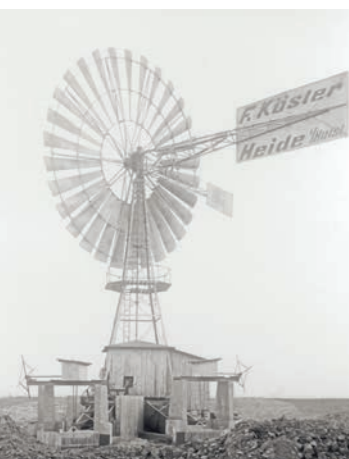
Fixed wind engine for generating electricity - innovation by KÖSTER- in the age of industrialization
