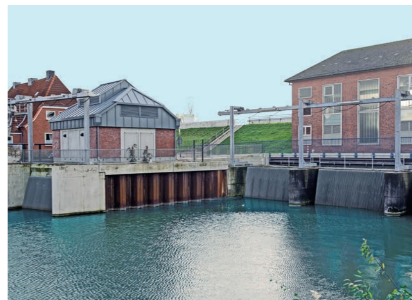
Pump Station Brunsbüttel-Nord VPH 1400 vertical Propeller pump, suspended 6,000 l/s 6.0 m 560 kW
