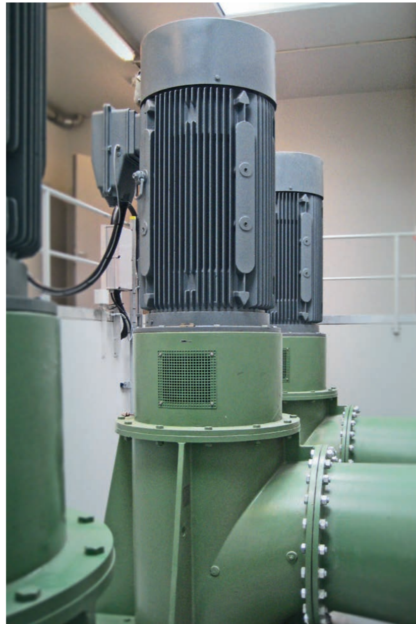
Pump Station Avedore Holme (Copenhagen, Denmark) VPH 800 vertical propeller pump, suspended 1,700 l/s 8.0 m 200 kW
