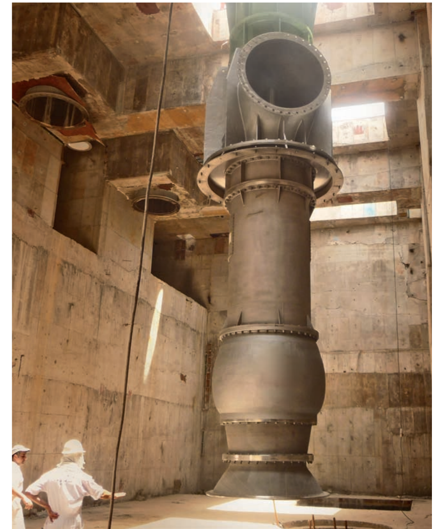
Dock pump on the Persian Gulf VKP 1400 vertical mixed flow pump 6,670 l/s 20 m 1,800 kW
