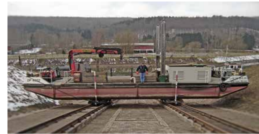
2009 Hannoversch-Münden Slipway system
