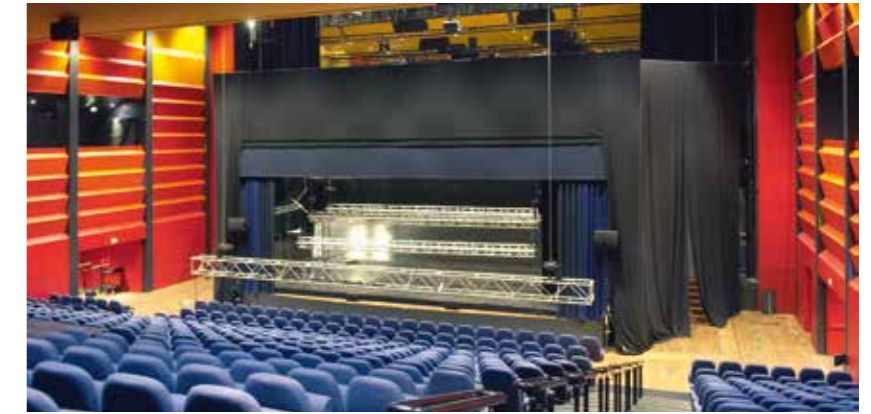
2003 Musikhuset Esbjerg Rigging system for stage decoration
